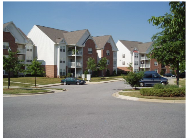
Covington Condominium Bowie, MD 96 units, 8 buildings
